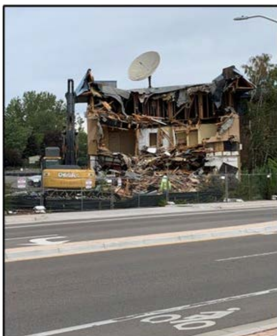
Hilltop House demolition
