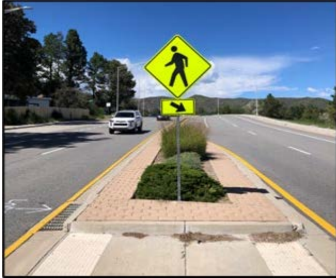
Installed new pedestrain crossings sign
