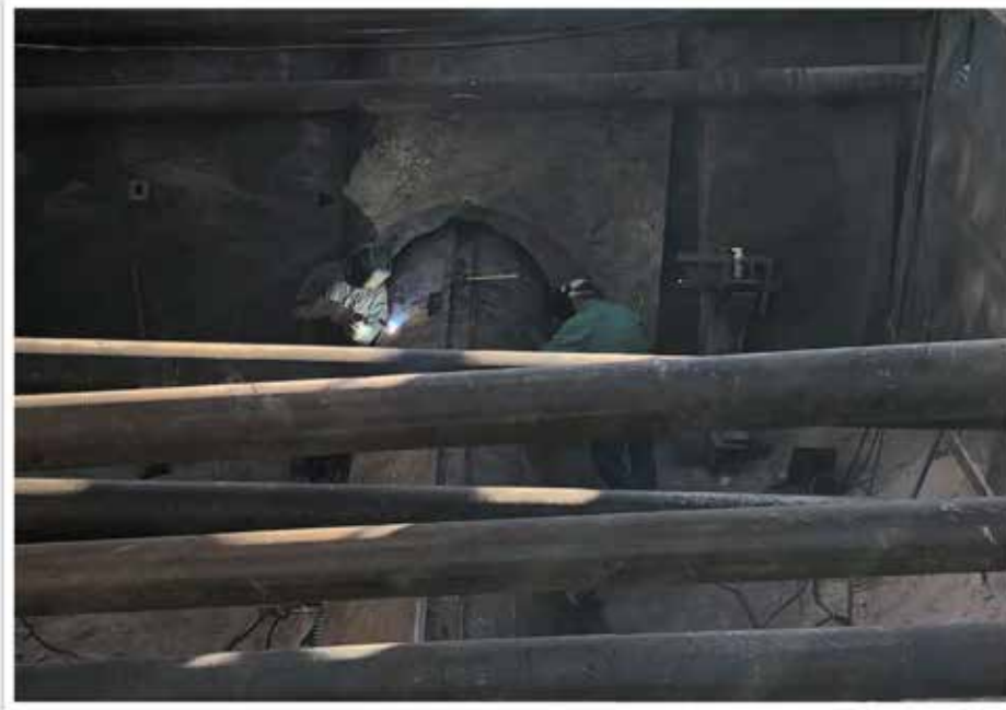
NM State Road 4 water main replacement.
