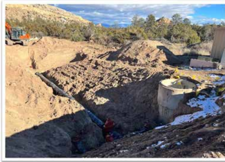
Bayo non-potable Tank Project
