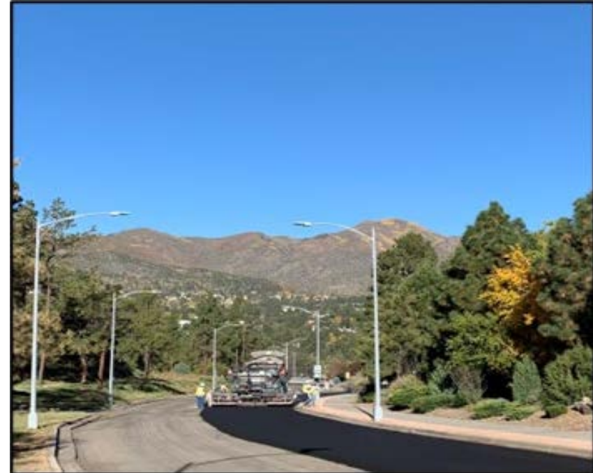
Completed the Canyon Road Roadway & Utilities Project
