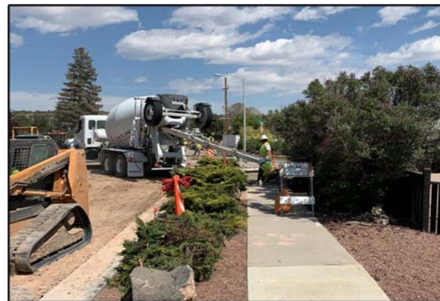
Completed Sherwood Blvd. Construction Project
