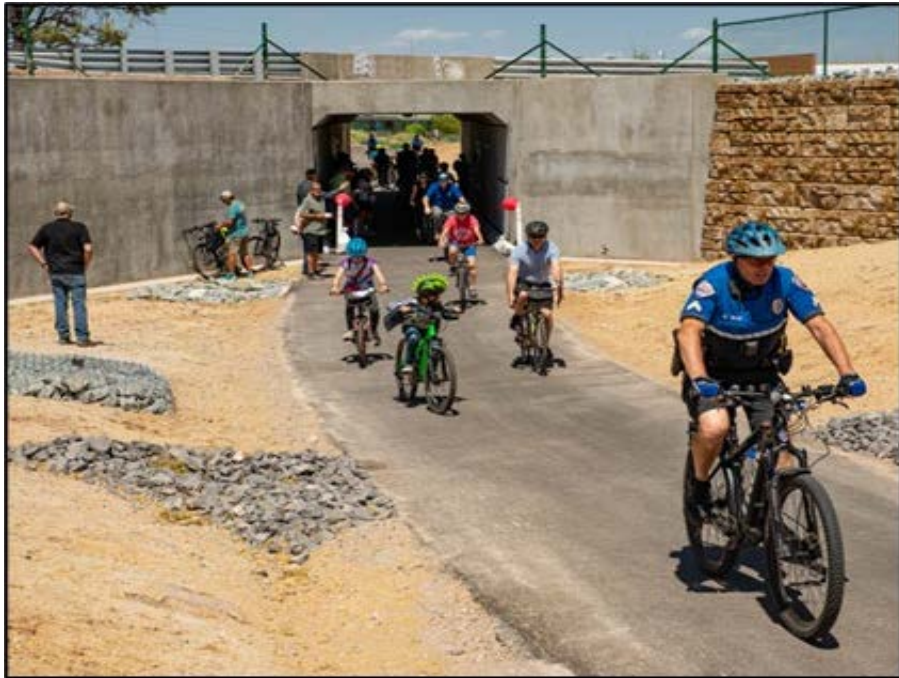
Completed Canyon Rim Trail Underpass
