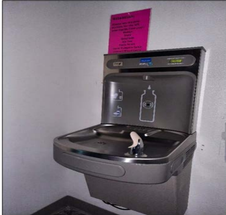
Crews installed water bottle filling stations
