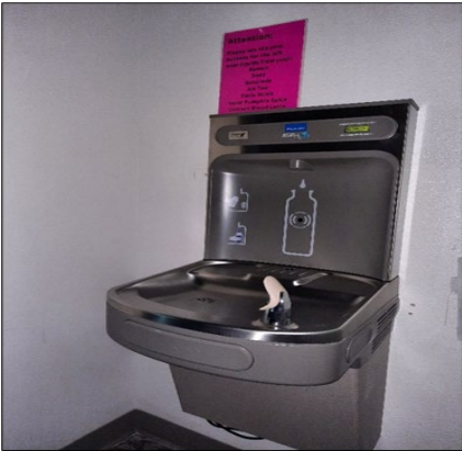
Crews installed water bottle filling stations
