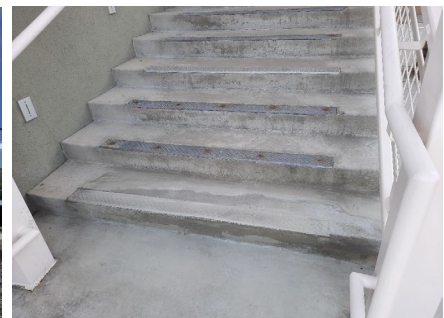
Golf Course Stairs and Snow Melt System Repair
