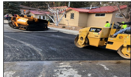
Crews repair asphalt
