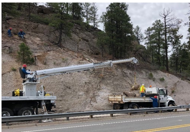
Crews remove rocks at North Mesa roundabout
