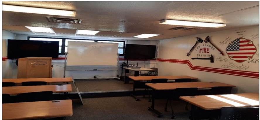
Crews painted the class room at Fire Station 2
