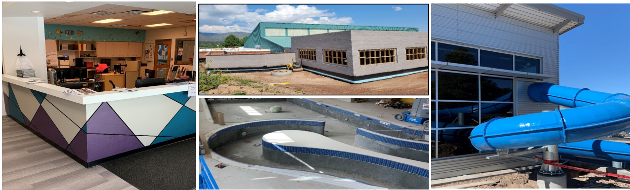
Construction of the Lesiure Lagoon and Aquatic Center remodel
