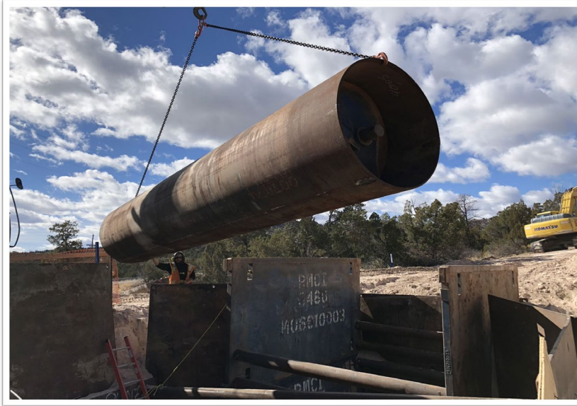
GWS crews work on the NM State Road 4 water main replacement.
