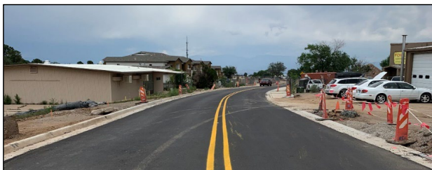
Contractor competes paving on DP Road
