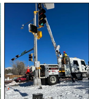
Crews repair street light Central Ave.
