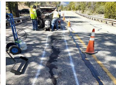
Pavement Preservation Project
