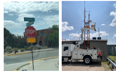
Signs fabricated and installed New rotating beacon at the Airport
