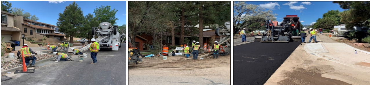
North Mesa Road & Utility Improvements - Casa de Oro
