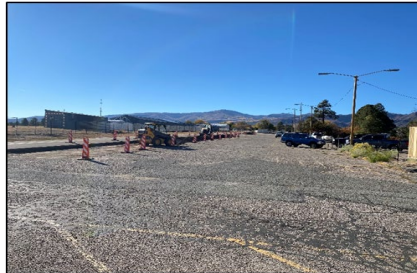
Storm Water Pollution Prevention Plan work at Los Alamos Airport
