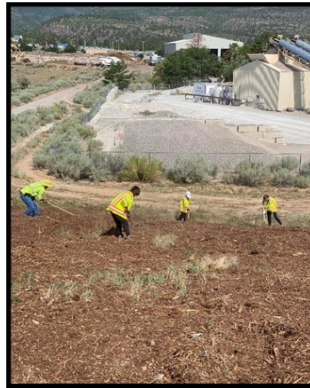
Y Corp volunteers stabilize landfill slopes
