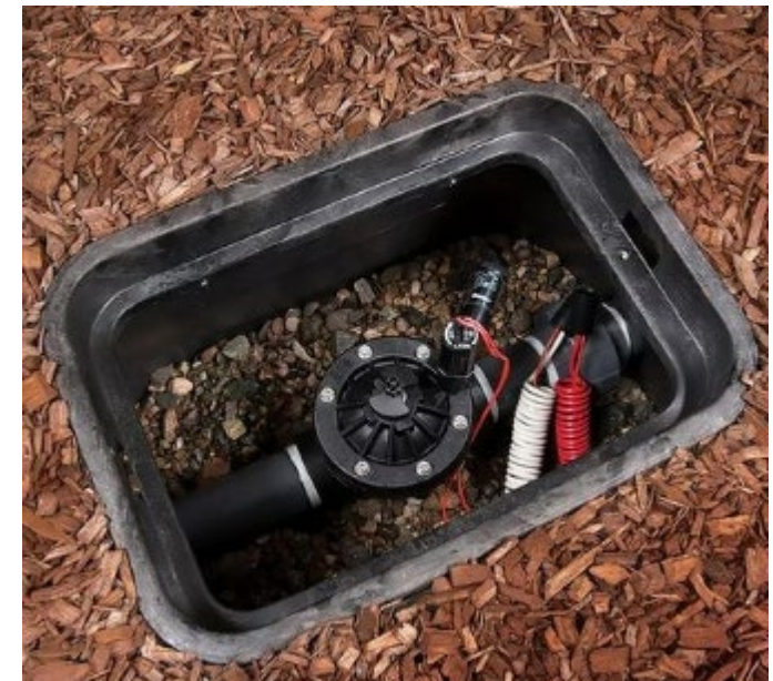
Irrigation Valve Box
