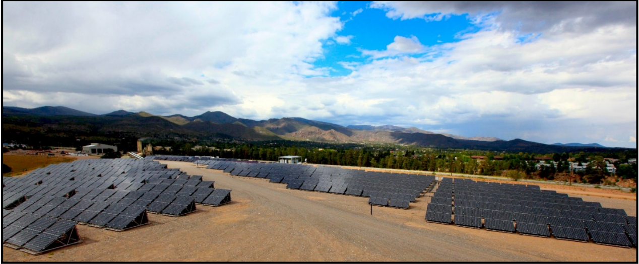
Figure 13: Photovoltaic array on the East Jemez landfill site
