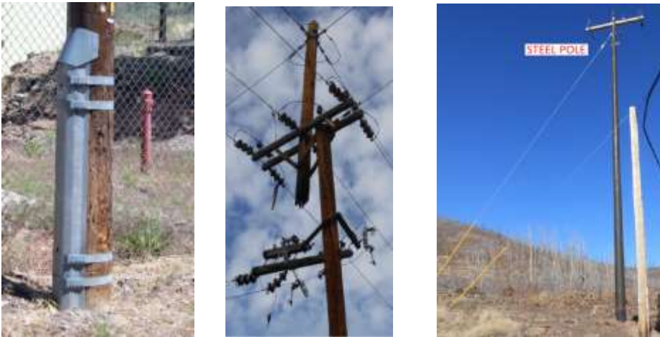
Figure 8B. Typical braced pole & backbone broken pole; & new Steel Pole
