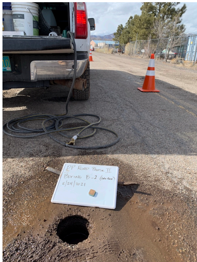
Boring B-2 After Coring
