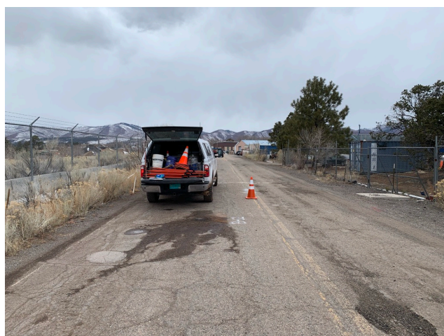
Boring B-2 After Completion
