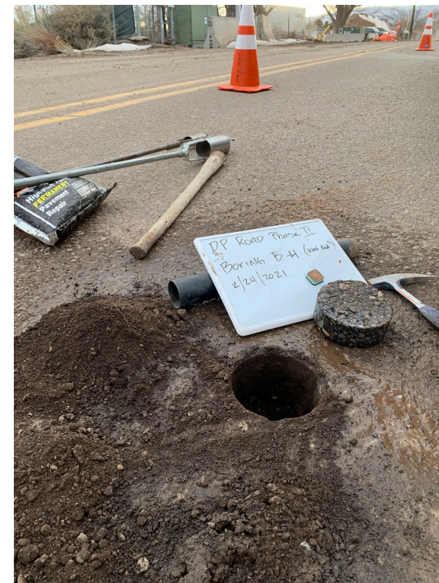
Boring B-4 After Coring
