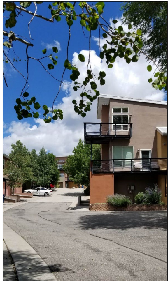
Narrow street at Canyon View Condo
