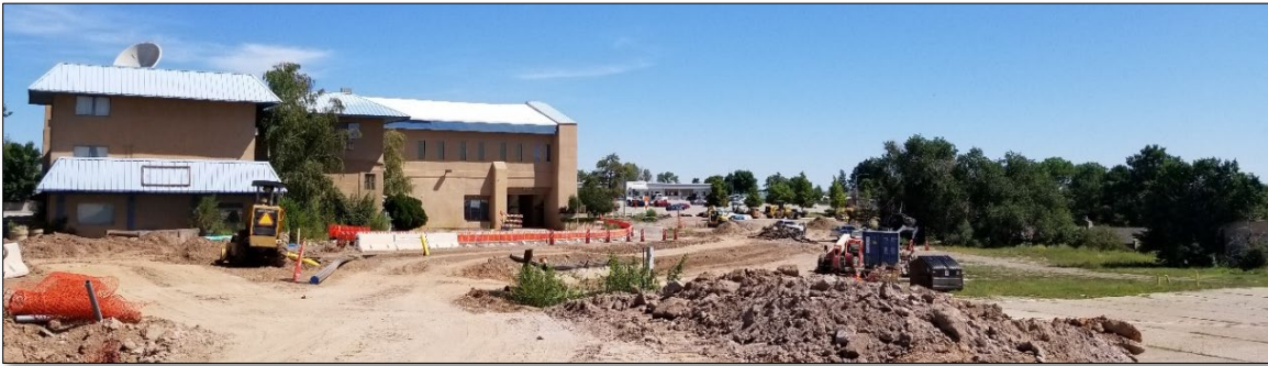
New Roundabout Construction (due for completion in 2021)
