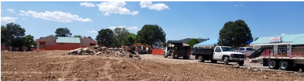
Removal of Condemned Buildings
