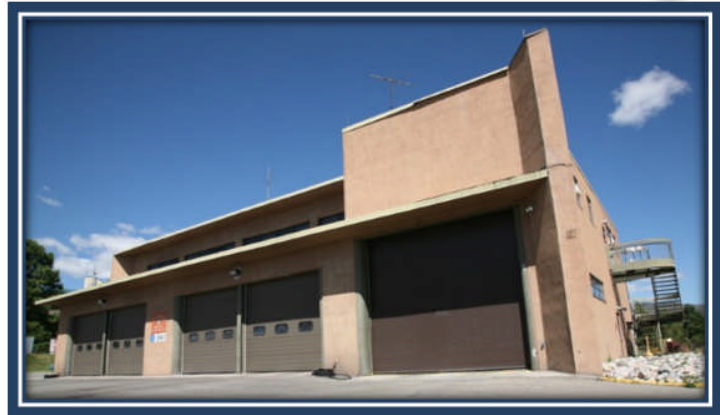
Picture 9 Fire Station 1 - West Jemez Road
