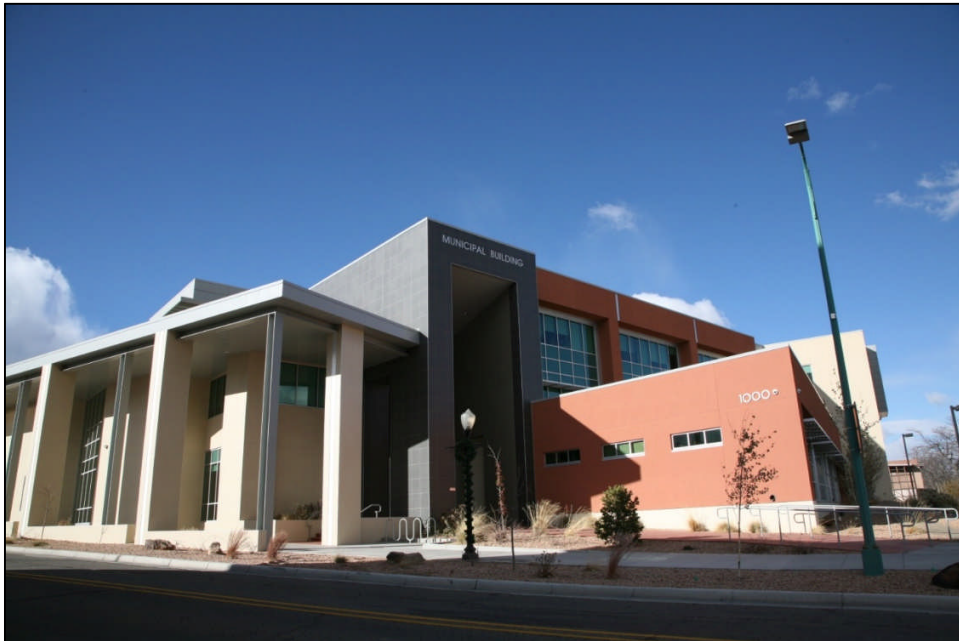
Los Alamos County Municipal Building
