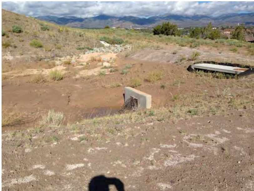
Figure 4.28. Airport Retention Pond Sediment
