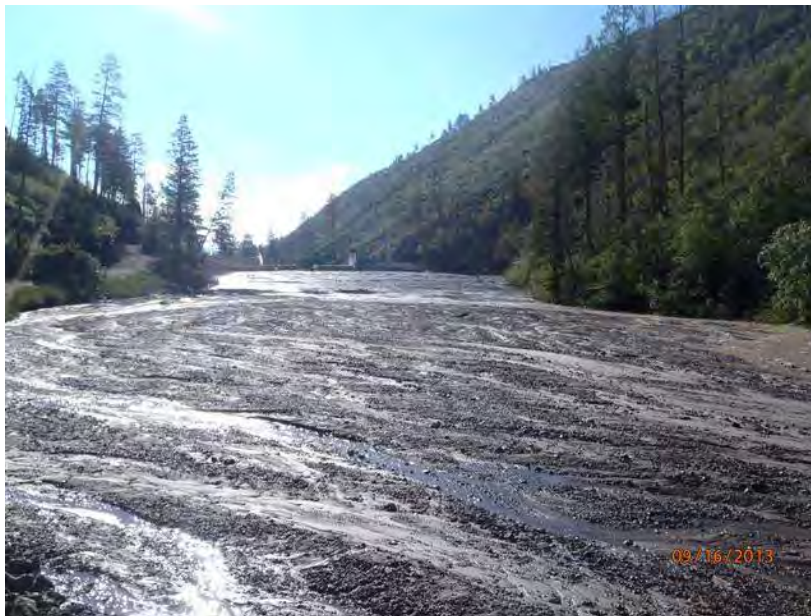
Figure 4.34. Sediment Filled Reservoir
