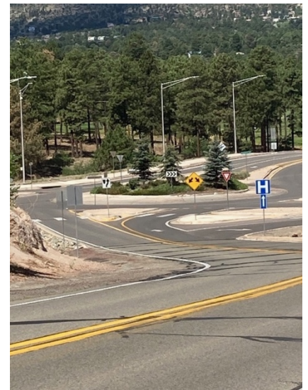
Roundabout between North and Barranca Mesas
