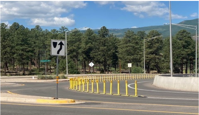
Bollards at Barranca/North Mesa roundabout.
