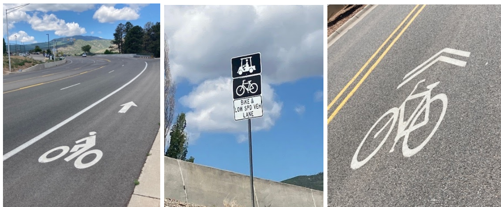
Bike lane and bike/low speed vehicle signage on Diamond Drive near Golf Course, sharrow in downtown Los Alamos
