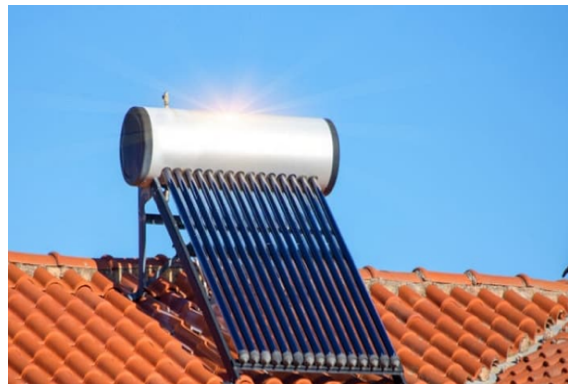
Example of rooftop solar water heater from Clean Energy Summit
