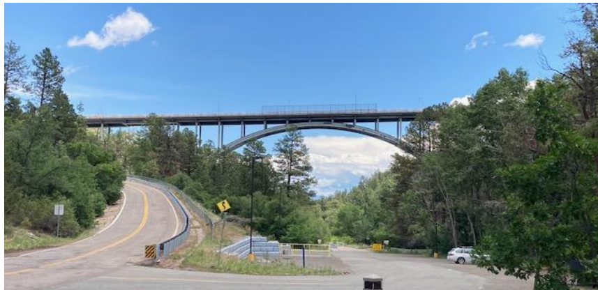
The Omega Bridge as seen from Los Alamos Canyon.
