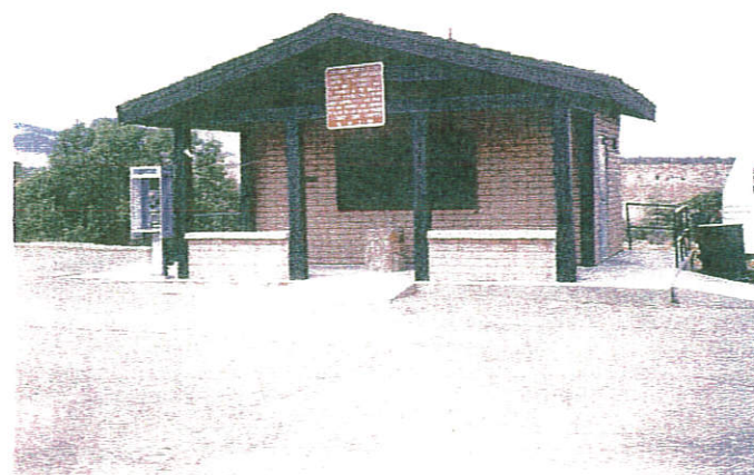
92 Paint restroom trim
