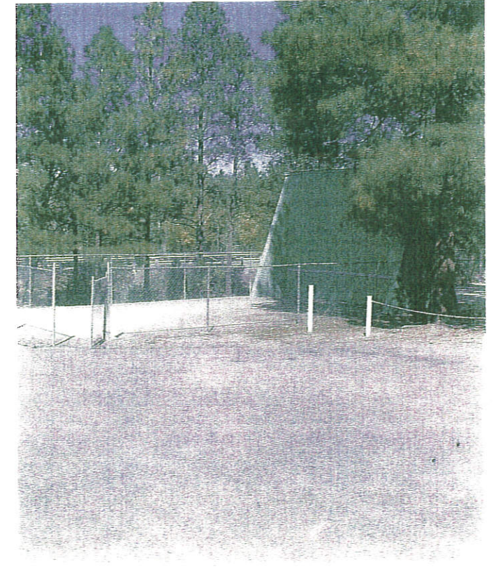
Patch/repaint ball wall
