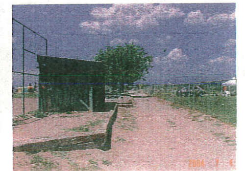
Repair wall and grade road
