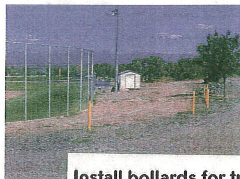
Install bollards for traffic control and parking
