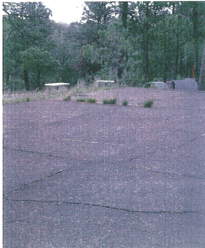
Restore basketball court
