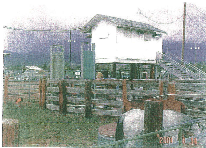
Repair and renovate crow's nest and chutes
