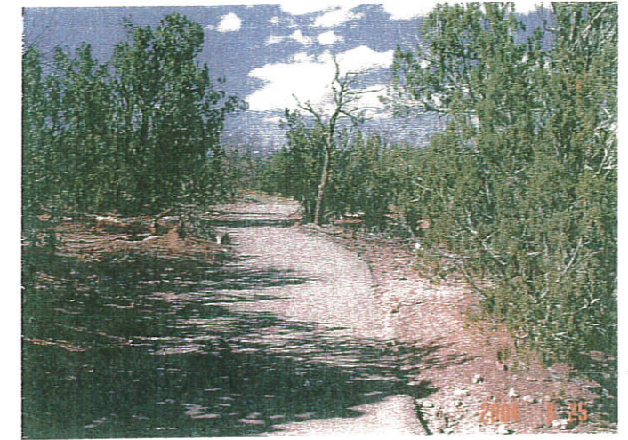
Repair trail system
