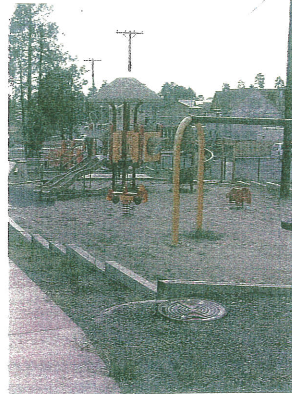
Replace sand w/new safety surface
