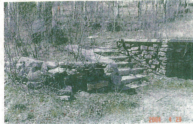
Raze and redo stonework
