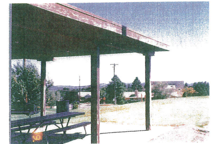
Repair and paint shelter
