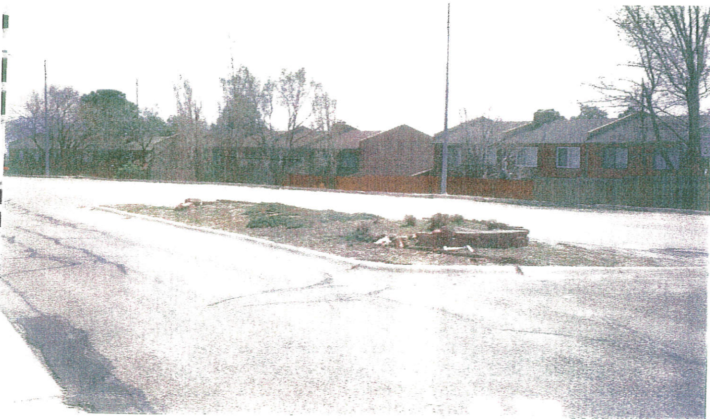
Traffic island to be removed
