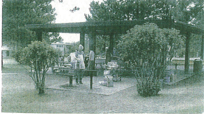
Repair and repaint shelter
