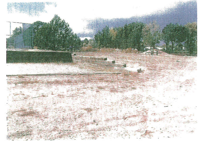
Replace failing walls
