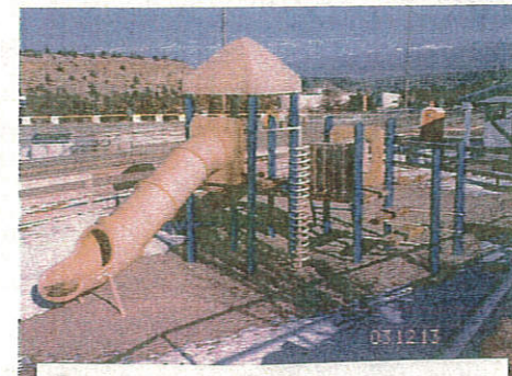
Replace safety surfacing
