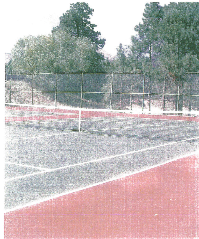
Clean courts regularly
