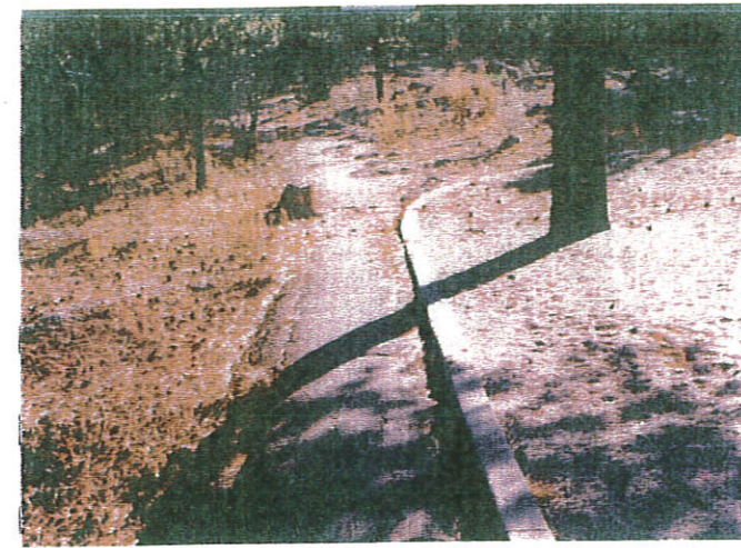
Repair trail route
