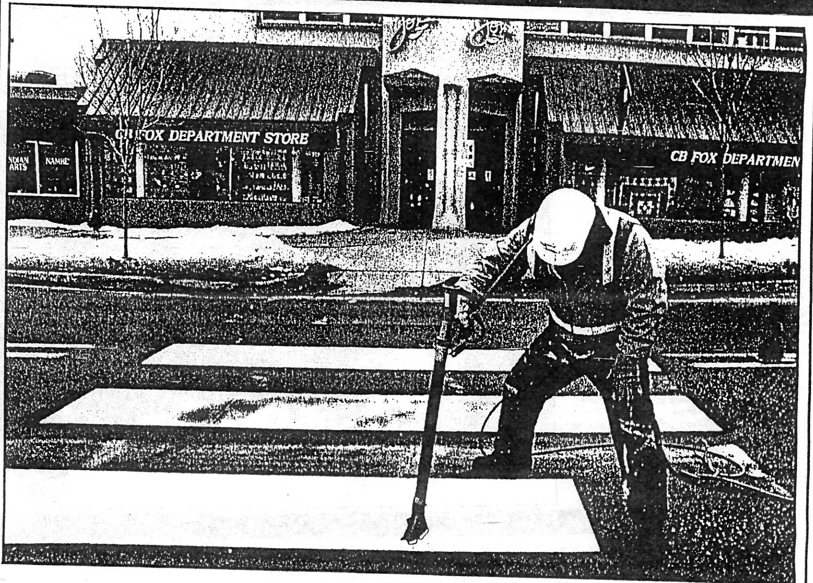
Downtown on Central Avenue, Los Alamos County employee David Rodriguez applies heat to thermo-plastic strips that will
