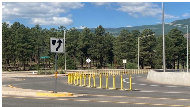
Bollards at the North/Barranca Mesa roundabout
