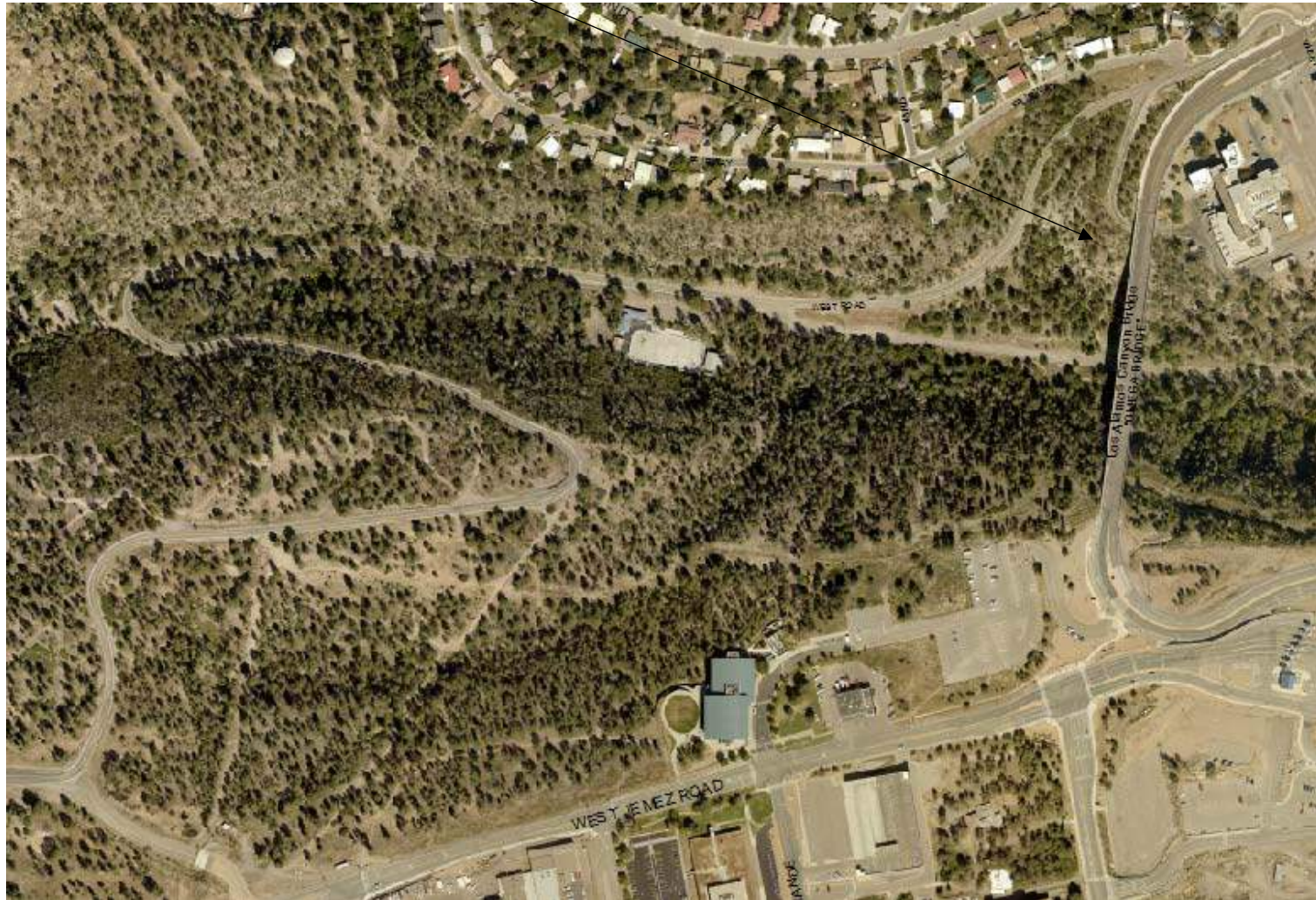
Approximate location – The remnant of the road is on LANL property and not open to the public.
