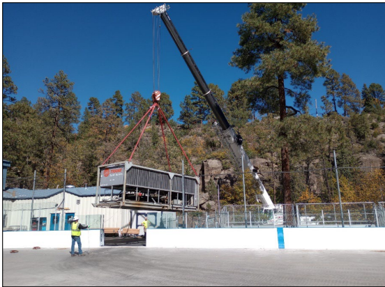
Installation of temporary chiller at the Ice Rink
