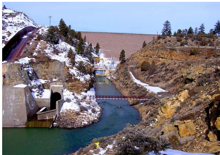
El Vado Hydroelectric Power Plant
