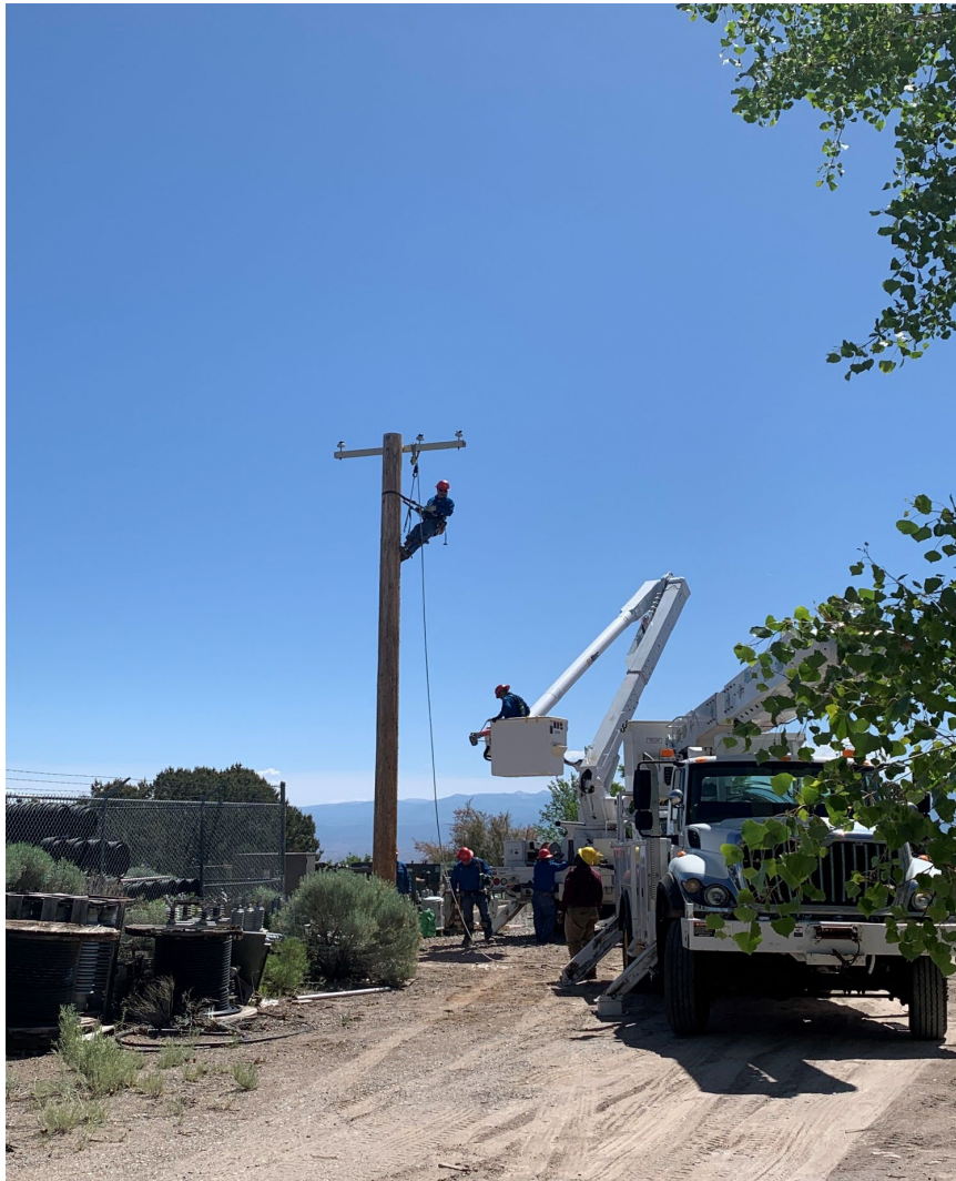
The Electric Distribution Division participates in overhead system safety training.
