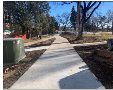
Urban Trail Construction Project
