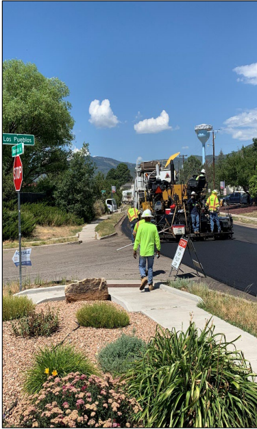
Barranca Mill & Overlay Project
