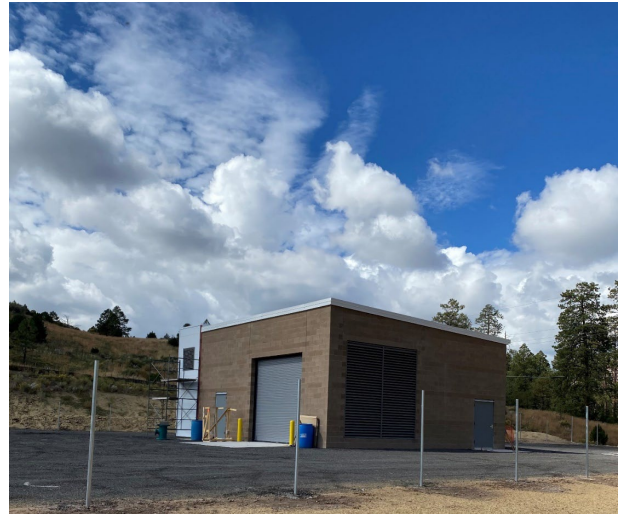
Construction of Otowi Well #2 was completed in FY2023. The total depth of the well is 2,310 feet, pumping from an elevation of 6,430 feet. The pumped water has a temperature of 84.4 degrees Fahrenheit.
