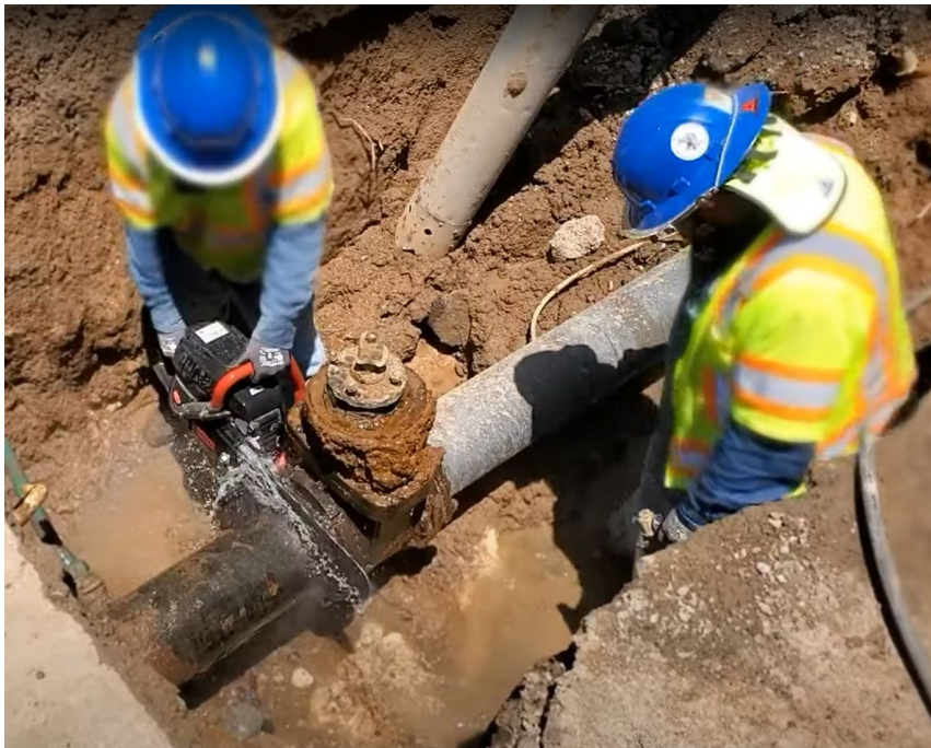
Water crews work on a water valve replacement.
