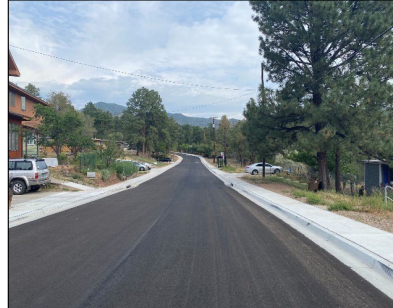
33rd/34th Streets Improvements
