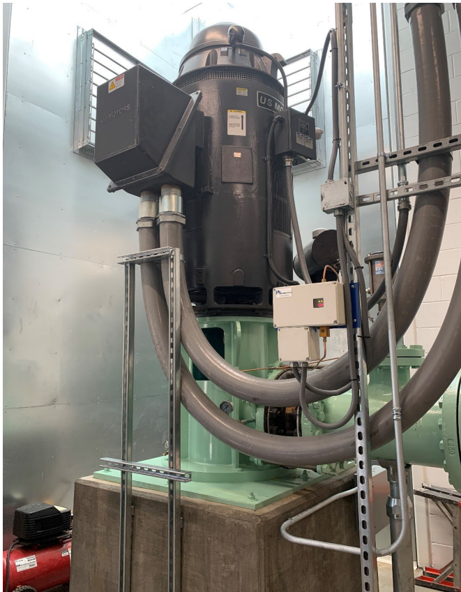
Construction of Otowi Well #2 was completed in FY2023. The total depth of the well is 2,310 feet, pumping from an elevation of 6,430 feet. The pumped water has a temperature of 84.4 degrees Fahrenheit.
