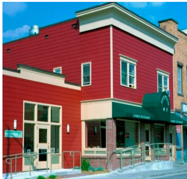
Facade improvement programs aid in the aesthetics of Town Center areas. This underutilized pair of commercial buildings in Hamilton, New York, was updated with a whole new color and look, including a new cornice, siding, windows, doors, awning, detailing and other signage.
