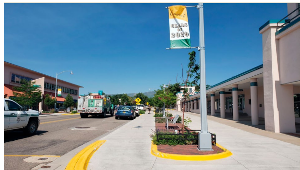
Existing improvements along Central Avenue
