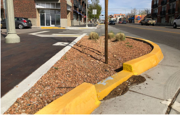
A curb cut to a bioswale allows stormwater to infiltrate through the soil naturally instead of being directly diverted to storm drains, Albuquerque, NM
