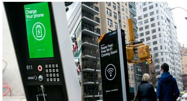
LinkNYC system supplies free public WiFi hotspots and charging stations.
