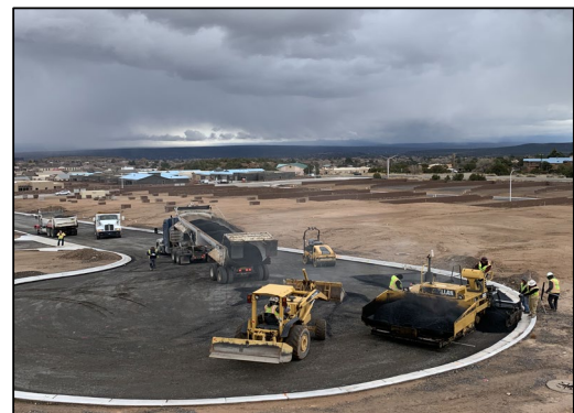
Paving at Mirador Subdivision
