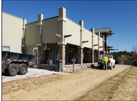
Golf Course Patio & HVAC Improvements
