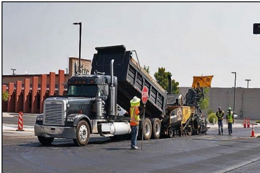
Paving on Trinity Drive
