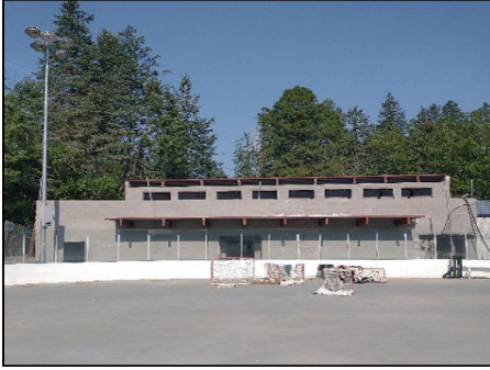
Ice Rink Improvements Project
