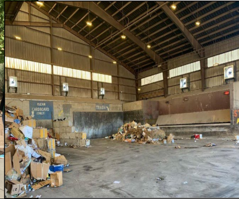
Transfer station ventilation system upgrade project
