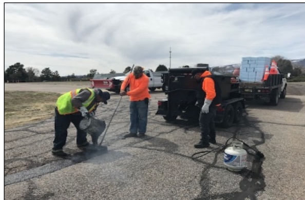
Pavement Maintenance at Los Alamos Airport
