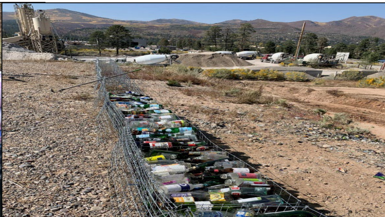
Landfill Slope Stabilization Project
