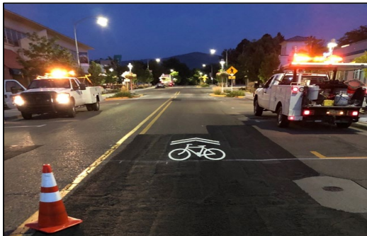
Crews replace pavement markings
