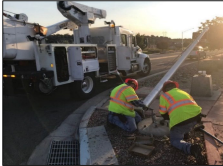
Crews repair a light pole due to an accident
