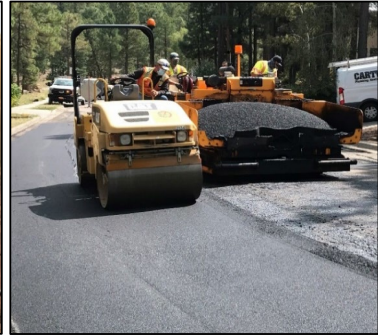
Repaving in the Ponderosa Estates
