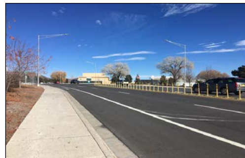
Diamond Drive Rehabilitation Project
