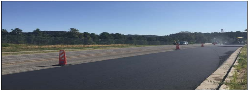
Diamond Drive Rehabilitation Project
