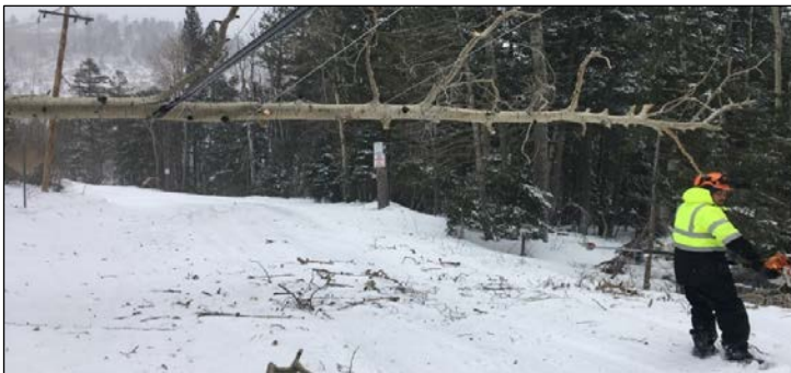
Cleanup work after wind and snow storm
