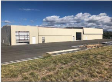
Airport Hangar Construction
