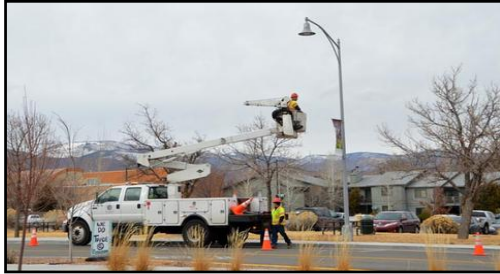
Electricians at work
