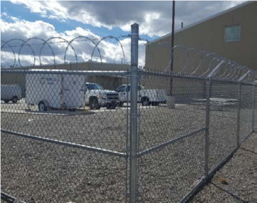
Installation of two new gates and barbed and razor wire at PCS to discourage after-hours access.
