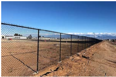
Perimeter Fence Project
