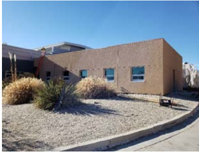
Fire Station 3 Renovations
