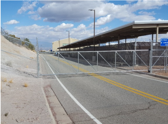
Installation of two new gates and barbed and razor wire at PCS to discourage after-hours access.
