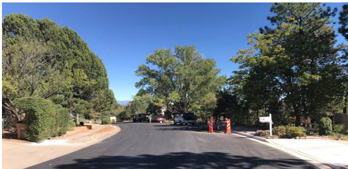
North Mesa Road Improvements Phase 2
