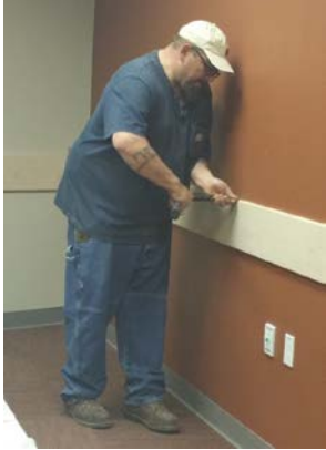
Tim Martinez installs chair guards in a conference room
