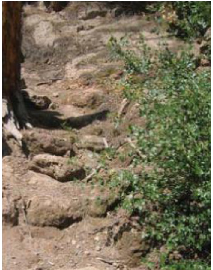
Improve stairs near 34th Street.
