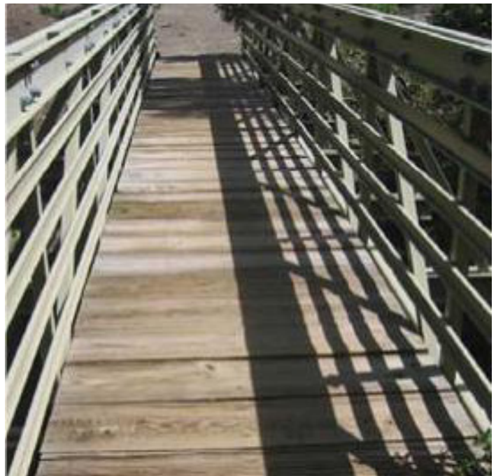
Replace bridge decking.
