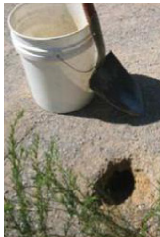
Monitor the condition of the road oil surface.
