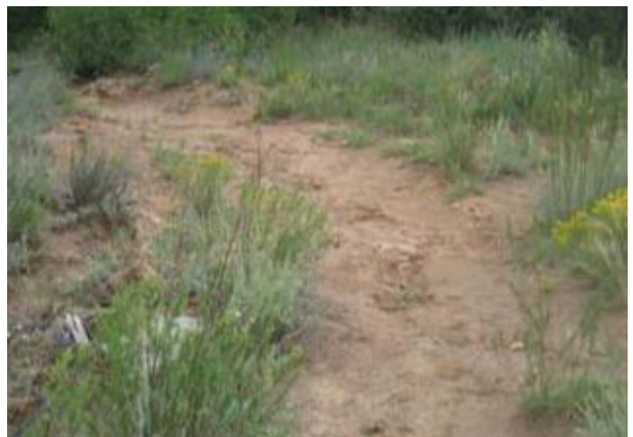
Monitor erosion at trailhead on Barranca Road.
