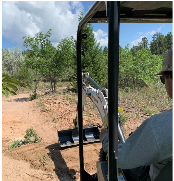
Building water bars at Quemazon trailhead.
