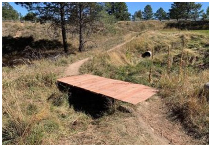
Monitor condition of bridges.
