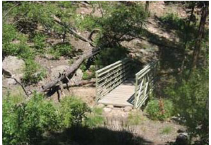
Monitor condition of bridge.
