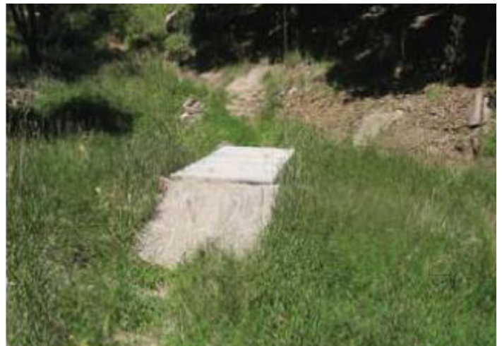
Monitor condition of bridge.
