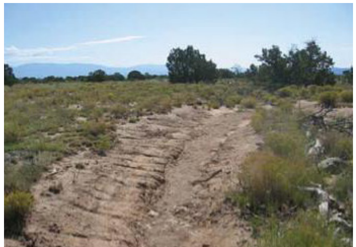
Move trail tread to stable surface at east end of trail.
