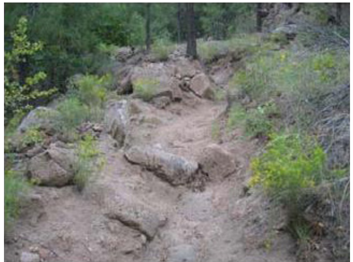
Move trail from deepening ruts to contour above.
