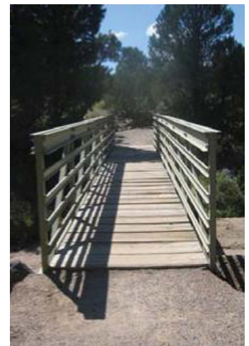
Monitor condition of bridge.
