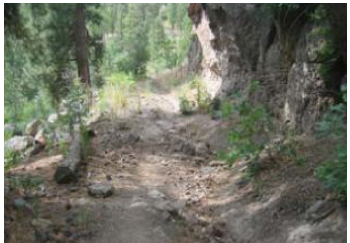
Fill in rut with small rocks to collect sediment.
