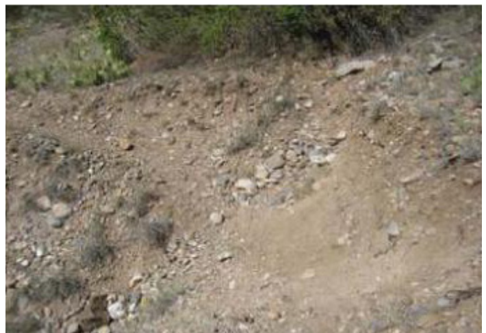
Reroute short section of trail at major drainages.
