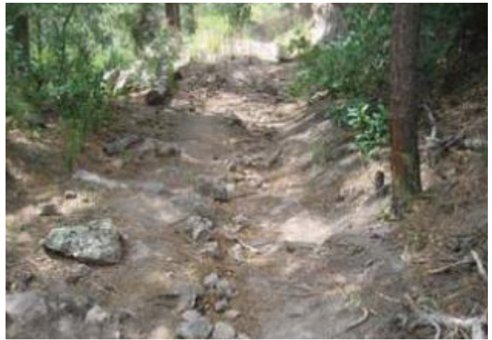
Monitor erosion on historic portion of trail.
