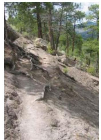
Extend retaining wall.
