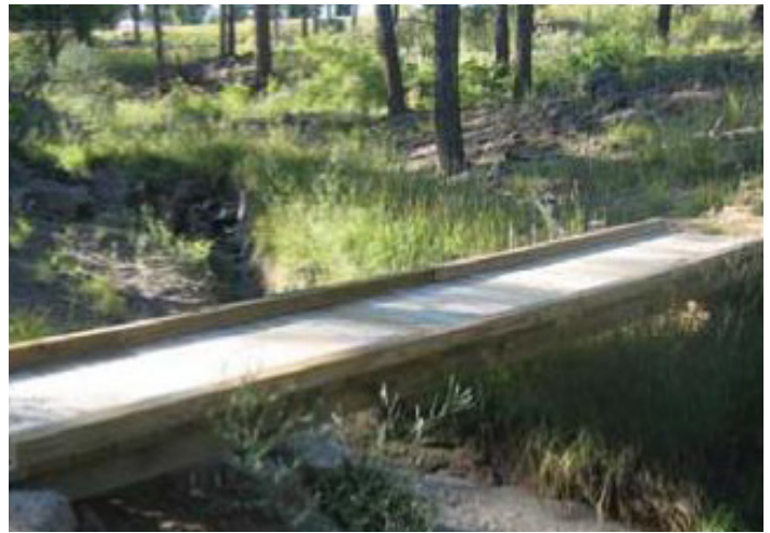
Monitor condition of the bridge near the roundabout.
