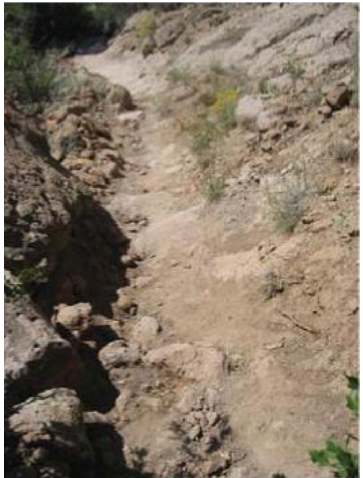
Repair stairs on middle switchback.
